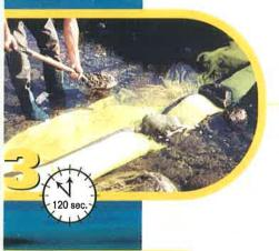
Push rocks to the rear and the job is done! The barrier is immediately created. Note the large rock at the bottom of the illustration, showing that the Water-Gate barrier can be used on any type of bottom.
