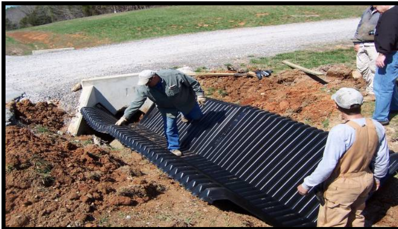
Ditch excavation, clean-out and site preparation for insertion of Smart Ditch
