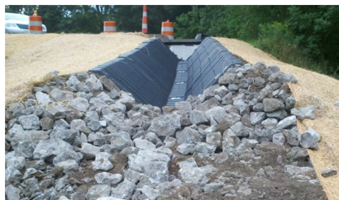
The old rip rap was repurposed to help dissipate stormwater flow at the end of the channel.
