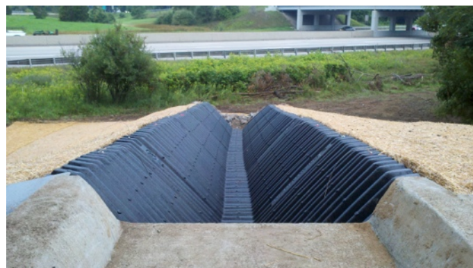
24" Trapezoidal SmartDitch replaced the old concrete and will not allow vegetation to grow and obstruct flow.
