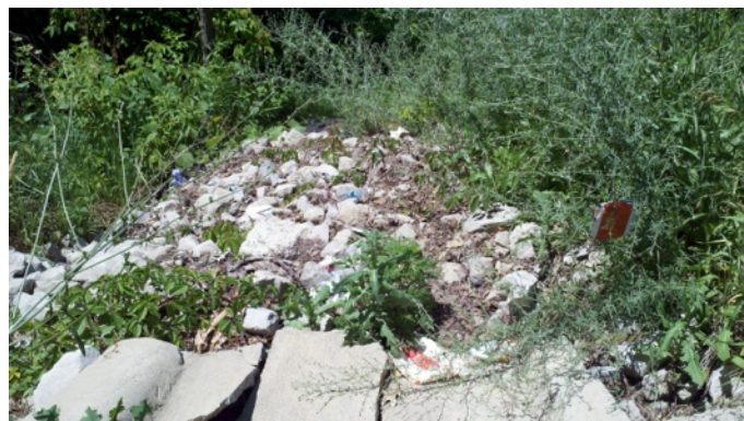
This overgrown, failed spillway was originally constructed of non-reinforced concrete and rip rap.
